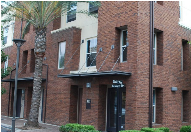
Brick finish wrapping the exterior corner
