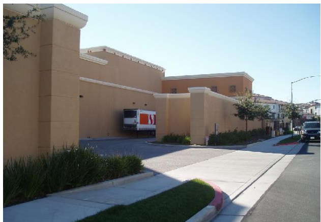
Screened loading area
