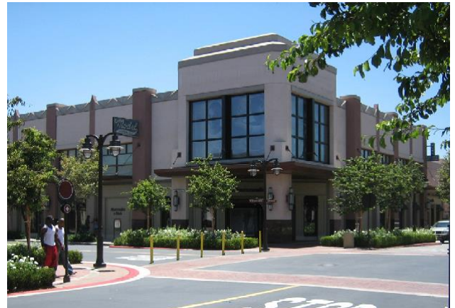
Prominent corner entry
