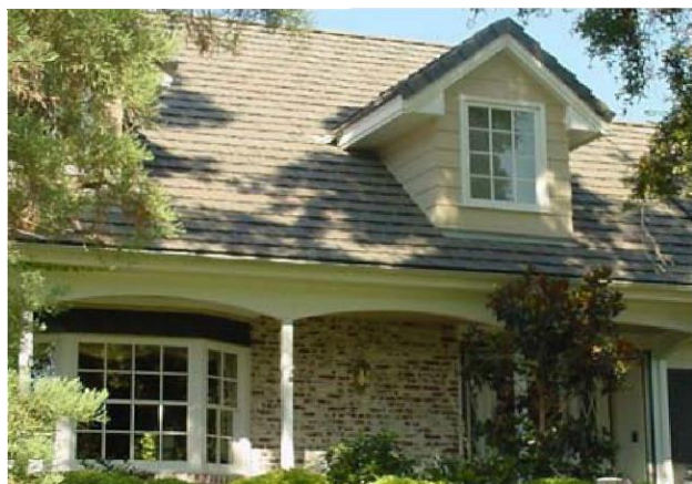
Balanced use of architectural details
