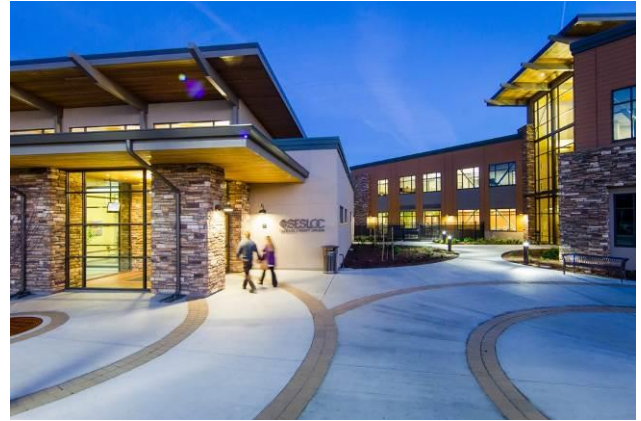
Lighting to enhance building features and walkways
